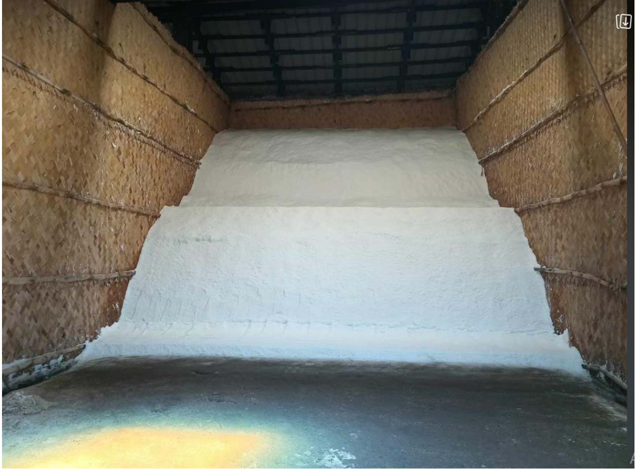
Figure 15. Documentation of Storage Area/ Facility
